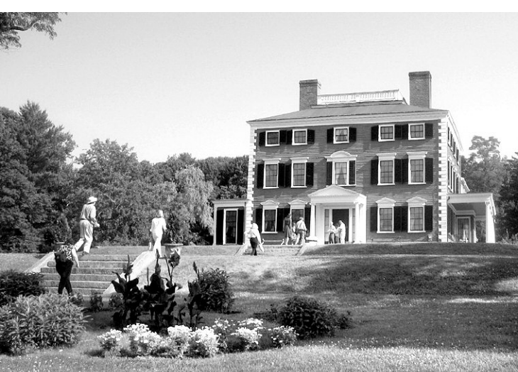
HNE's 1740 Codman House in Lincoln, Massachusetts, faced demolition in the mid-19th century but was saved after public outcry over the 1863 razing of John Hancock's 1737 Boston mansion.
