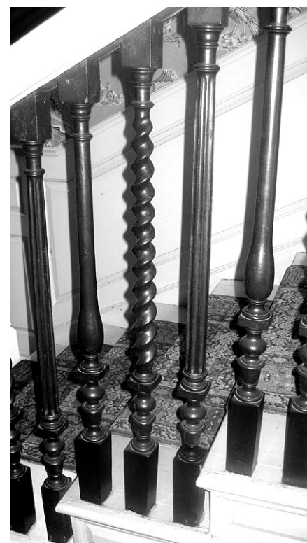
Virtuoso carving and lathe work are visible throughout the Langdon House. One motif is the three styles of turned balustrades repeated up the main staircase.
