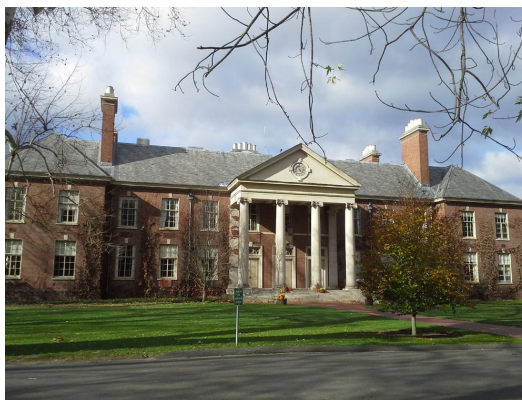
The brick Neoclassical main school building of Deerfield Academy overlooks the town's Old Main Street. The school was founded in 1797 and prepared many New England boys for productive lives in the new republic. Frishman photo.
